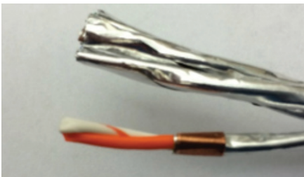
Figure 36: Removing the foil edge
