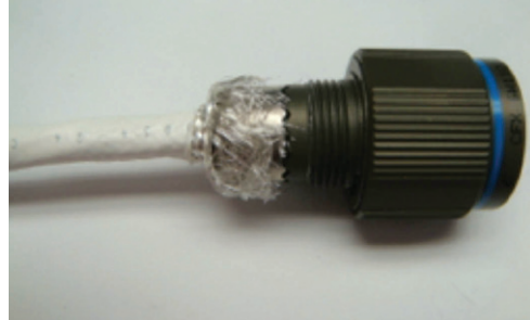
Figure 25: Trimming the excess braid material
