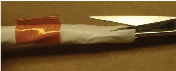
Figure 53: Cutting the outer jacket
